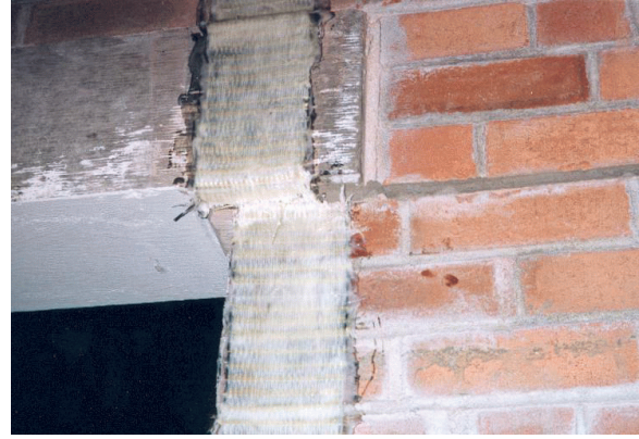
Figure 10. Tyfo strip failed in shear.
